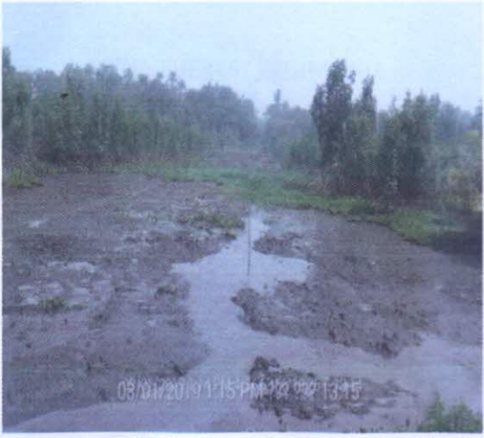
SPILL POINT BEFORE EXCAVATION: fig1
