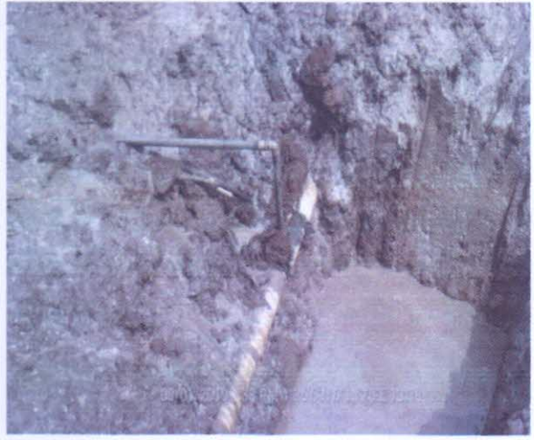
SPILL POINT AFTER EXCAVATION: fig2
